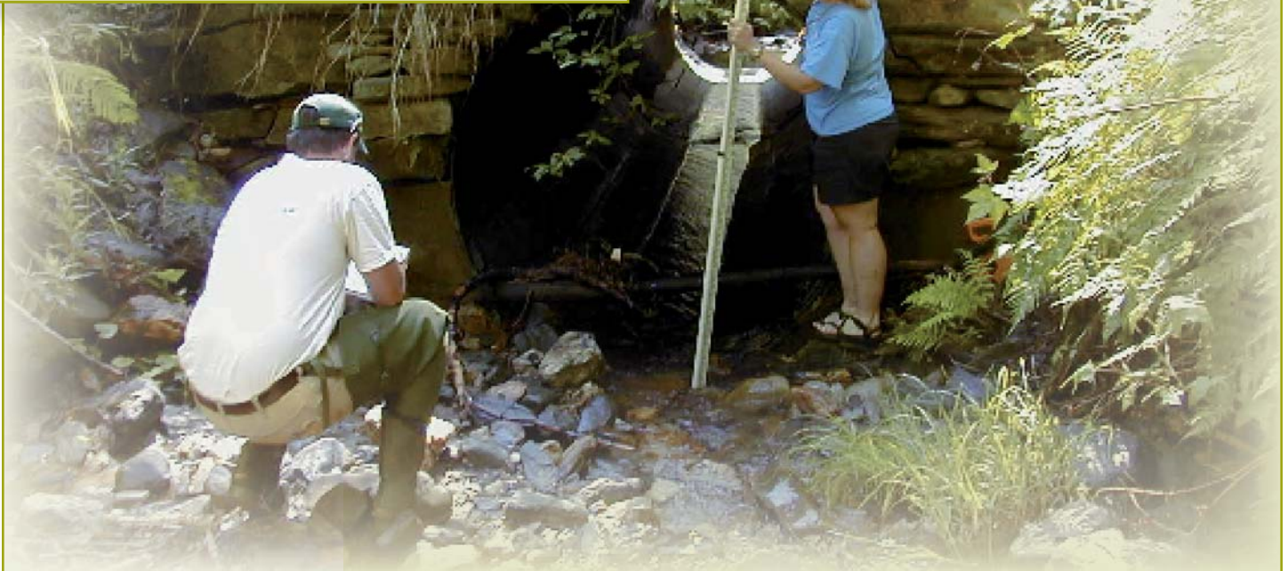
Culvert assessment/C. Alexander
