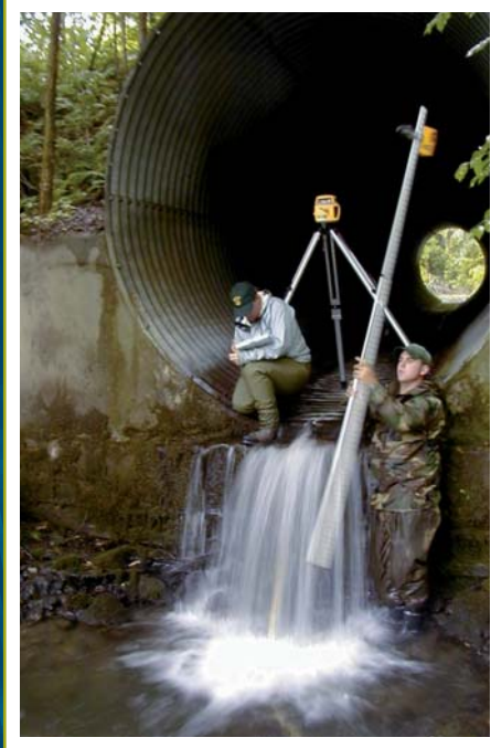
Culvert assessment/C. Alexander
