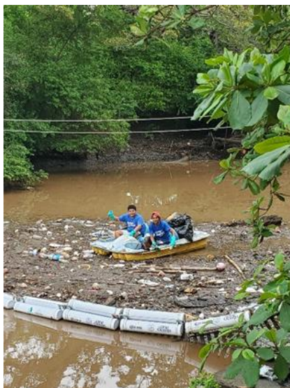
Figure 11: River intercept system at work to remove plastics on the El Tunco River.
