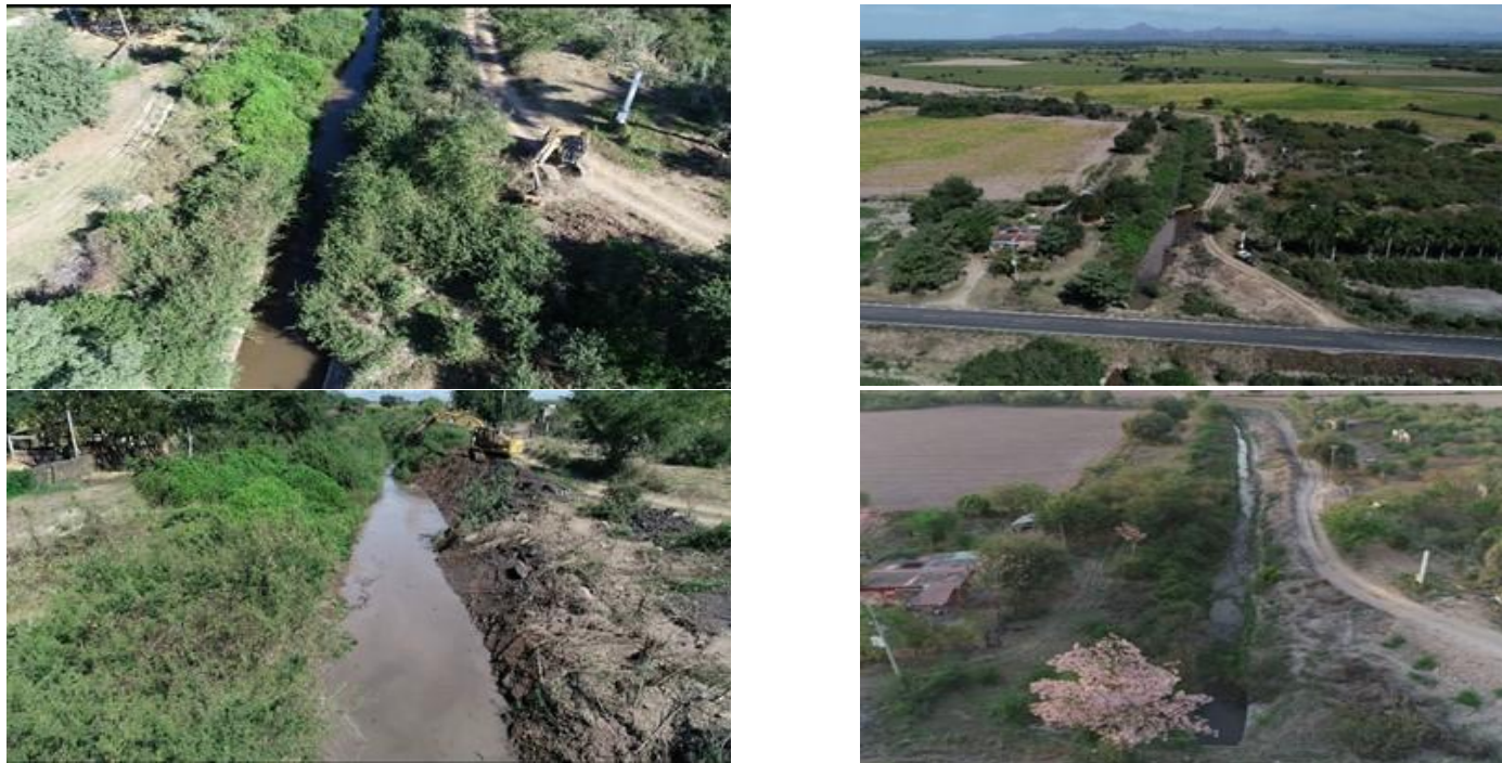
Figure 32: Photos showing the start and progress of the cleanup of 8.7 miles of the Viejo River channel.
