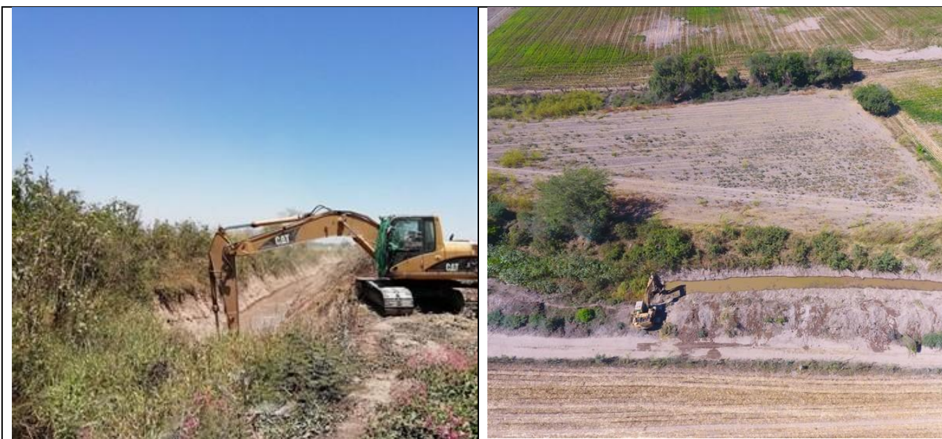
Photo of hydraulic excavator removing sediment and dead wood that obstructs the flow of water in Río Viejo
