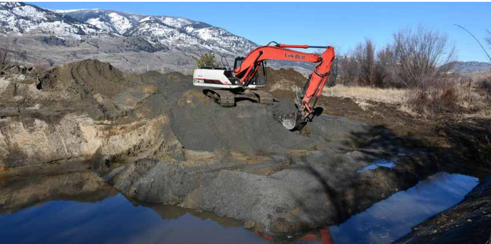
Wetland construction underway on the Winters property, southern British Columbia. Ducks Unlimited Canada
