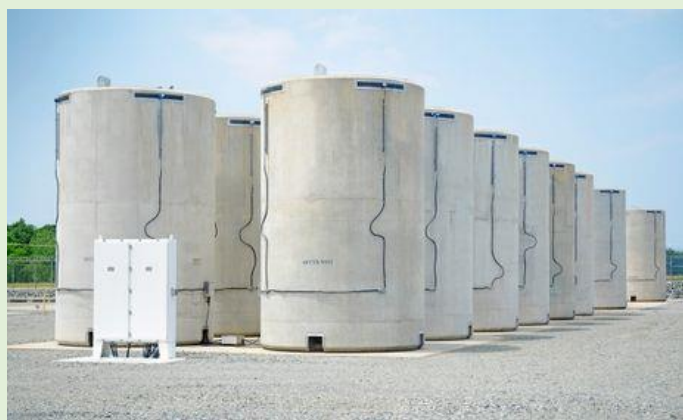
Dry Cask Storage System 300
