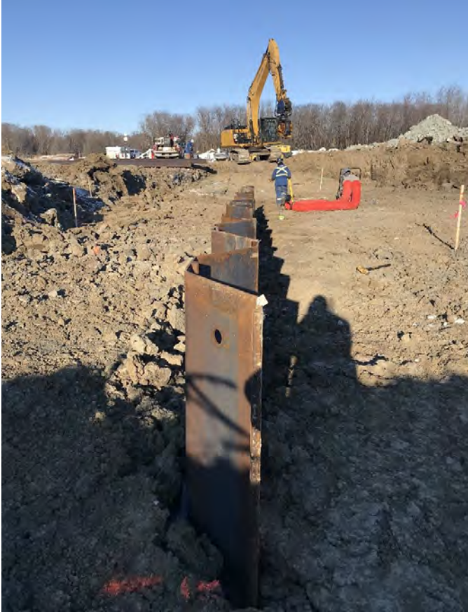
Birch Lake outlet rebuild. Ducks Unlimited Canada
