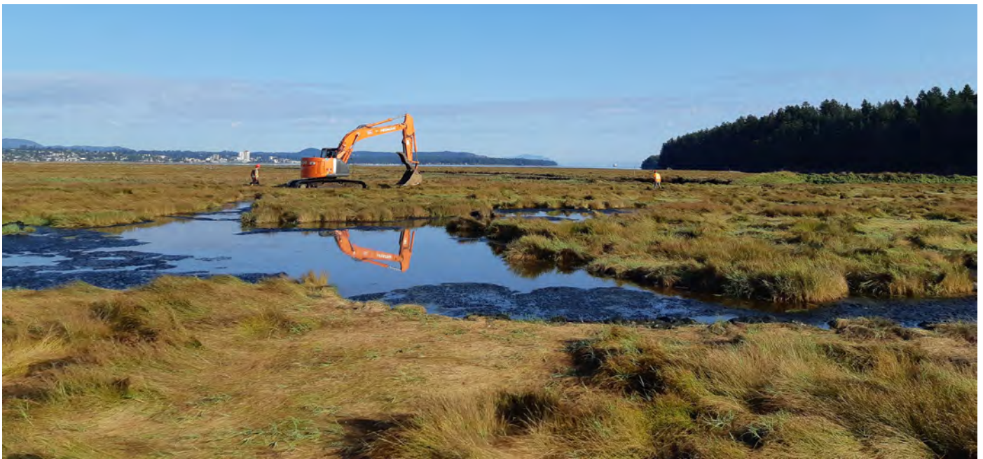
Restoration underway at the Nanaimo River estuary. Curtis Rispin, NTBC/WCCLMP
