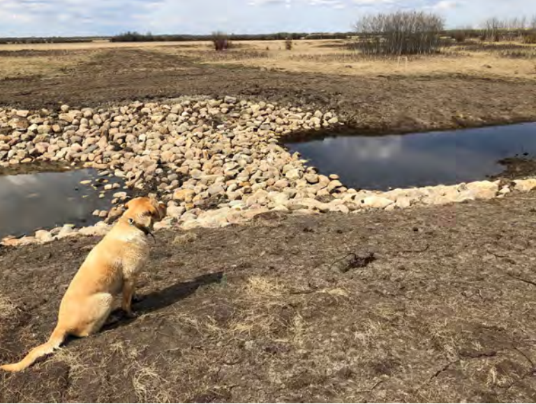
Control structure built to restore wetlands in the Alberta project.
