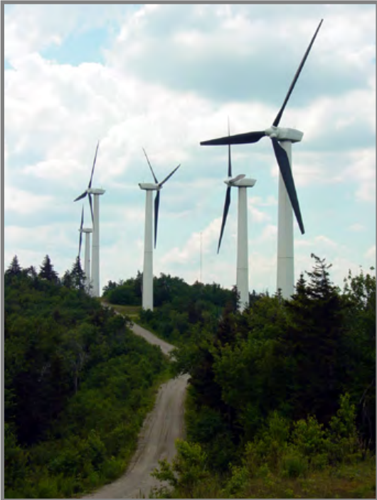
Southern Vermont wind farm - Courtesy VFWD
