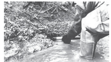
Dig pocket at water line
